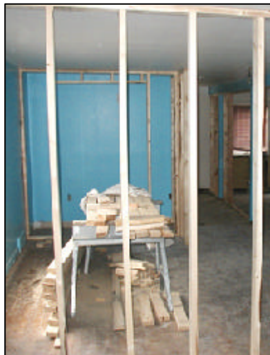
Remodelling inside the former Salvation Army building
